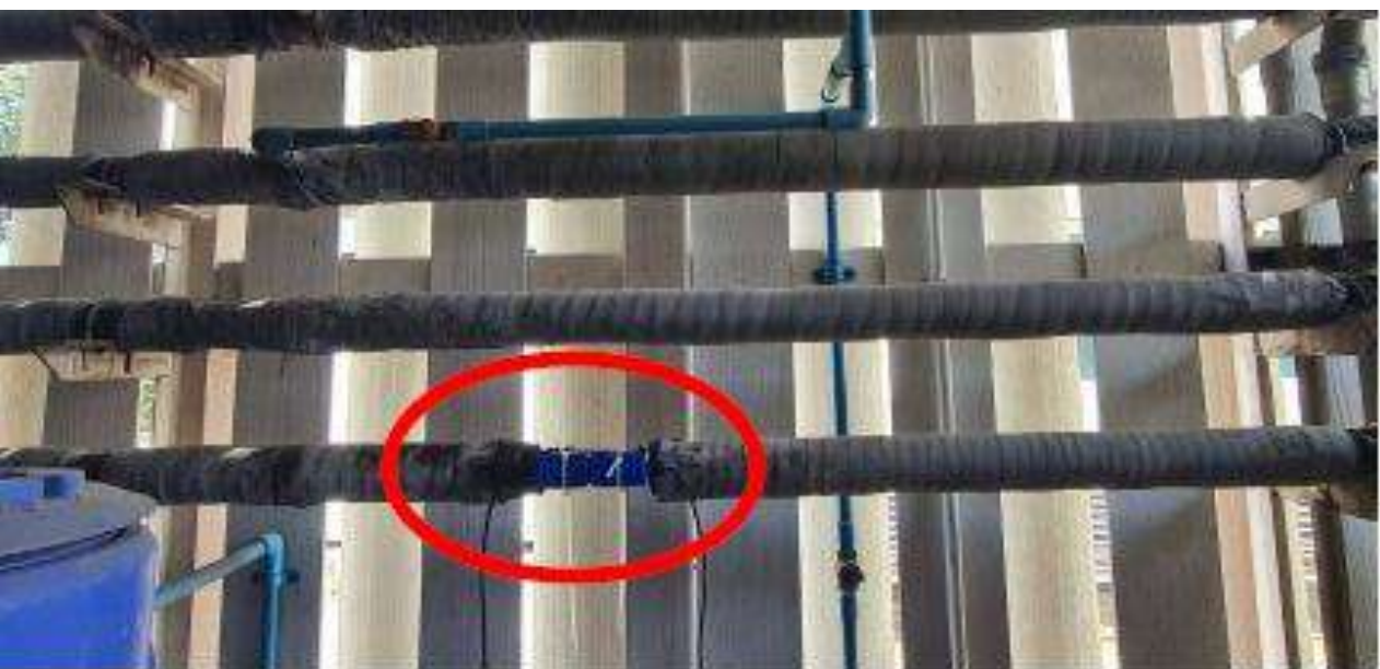
Chilled water flow rate (GPM)
